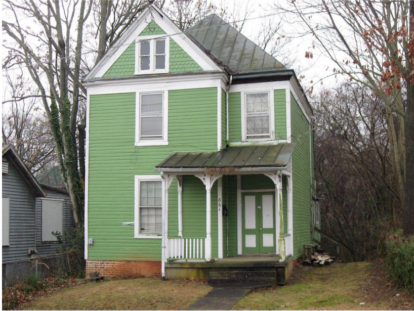
861 Pine – Façade (north)
