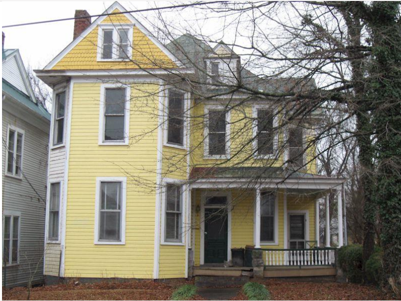
238 Jefferson Avenue – Façade (northeast)
